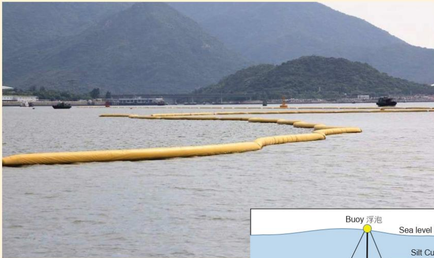
淤泥屏障 Silt curtains
