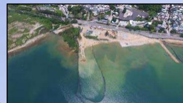
Silt curtain at Lung Mei Beach, May 2018
