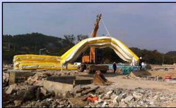
Handling of the silt curtain
